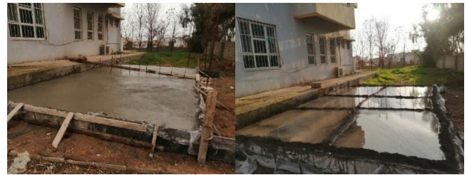
Figure (5) casting the concrete slab procedure
